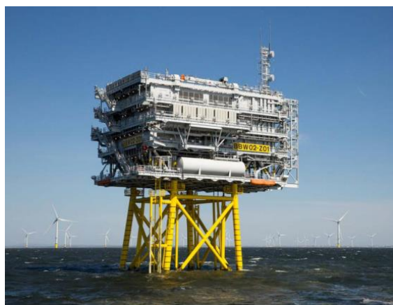
Fig. 3. View of platforms with HVAC Collector Stations.
