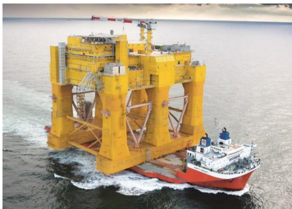
Fig. 10. View of the DolWin-2 offshore platform with the HVDC Converter Station , with a complete set of devices manufactured by ABB , power value 924 MW (platform weight approx. 20.000 tons)
