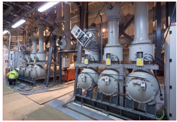
Fig. 11. View of GIS 400 kV type ELK-3 installed on the DolWin-2 platform : HVDC Converter Station with a power value of 924 MW , protected autotransformer and converter devices against short circuit current , generated in large Wind Farm Complex.
