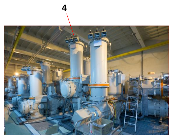
Fig. 8. Example of multi-bays gas insulated switchgear type ELK-04 , installed in the high-power HVAC Collector Station offered for 66 kV (busbar current 4000 A, circuit current 63 kA/3s).
