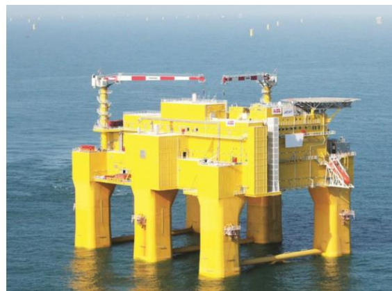
Fig. 10. View of the DolWin-2 offshore platform with the HVDC Converter Station , with a complete set of devices manufactured by ABB , power value 924 MW (platform weight approx. 20.000 tons)
