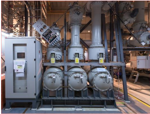
Fig. 11. View of GIS 400 kV type ELK-3 installed on the DolWin-2 platform : HVDC Converter Station with a power value of 924 MW , protected autotransformer and converter devices against short circuit current , generated in large Wind Farm Complex.
