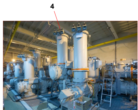
Fig. 8. Example of multi-bays gas insulated switchgear type ELK-04 , installed in the high-power HVAC Collector Station offered for 66 kV (busbar current 4000 A, circuit current 63 kA/3s).
