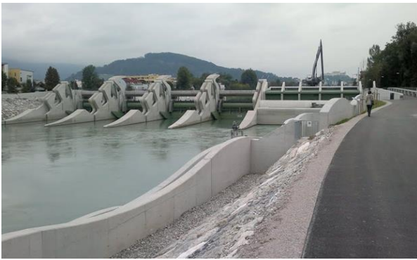
Fig.1 The Sohlstufe Lehen HPP on the Salzach River in Austria. View from the downstream
