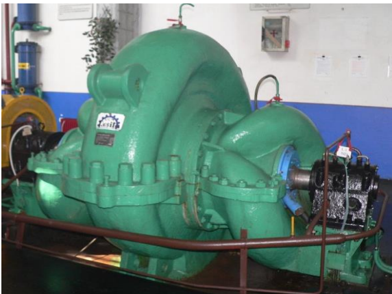
Fig.1 One single stage double-flux storage pumping unit
