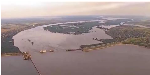
Fig. 4 Kakhovka HPP. Flooding of the off-site territories as a result of destruction
