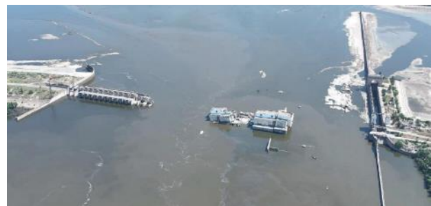
Fig. 3 View of the destroyed Kakhovka hydro development
