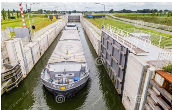
Fig. 4 Lock Empel in the province of North Brabant, in the south of Netherlands. View from the side of the lower gate
