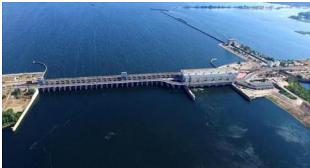
Fig. 1 Kakhovka HPP before its destruction. View from the downstream.
