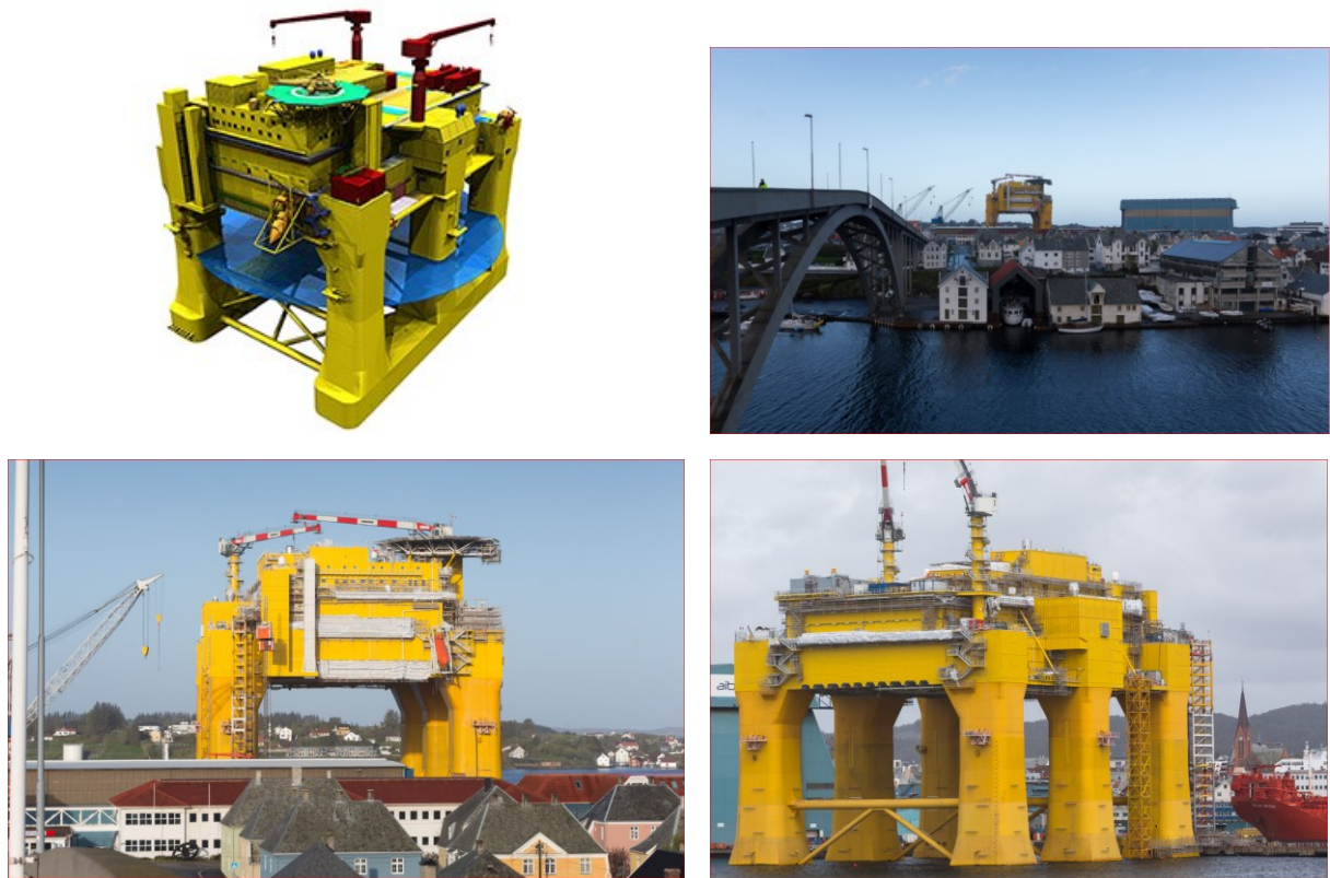
Fig. 10. View of the DolWin-2 offshore platform with the HVDC Converter Station, with a complete set of devices manufactured by ABB, power value 924 MW (platform weight approx. 20.000 tons).
