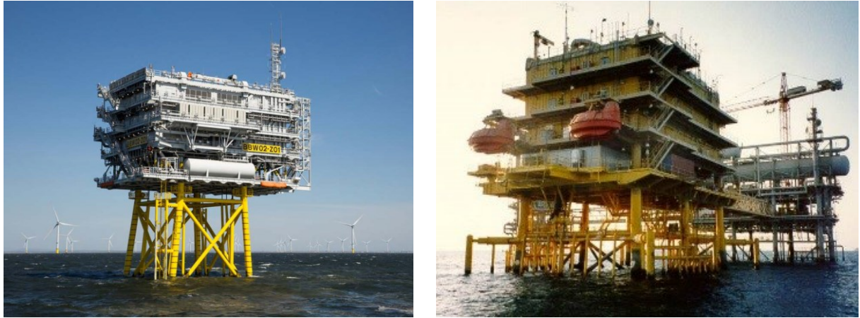
Fig. 3. View of platforms with HVAC Collector Substations.
