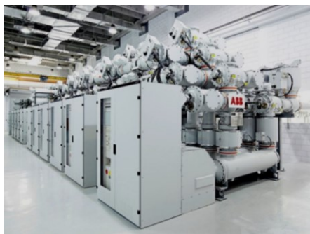
Fig. 7. Configuration of the complete 220kV bay SF6 insulated type ELK-14/300, used in offshore HVAC High Power Collector Substations.
