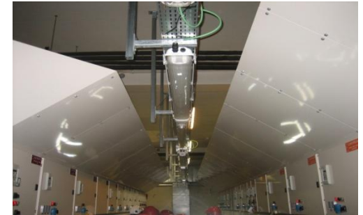
HV switchboard with deflector (internal arc)
