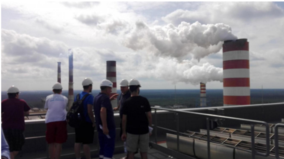
On the rooftop of B11, the latest power unit of the Koźienice Power Station – capacity of 1075 MW
